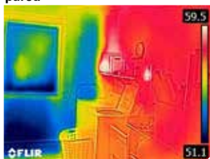
Pared exterior sin aislar
